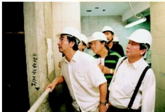
The weekly inspection team is inspecting the lift shaft guard-rails
