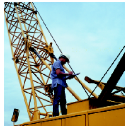
Mechanic is conducting a weekly check up on the mobile crane
