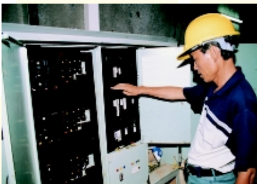
Inspecting electrical installations prior-to-work
