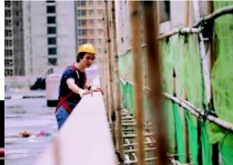
Inspecting scaffoldings prior-to-work
