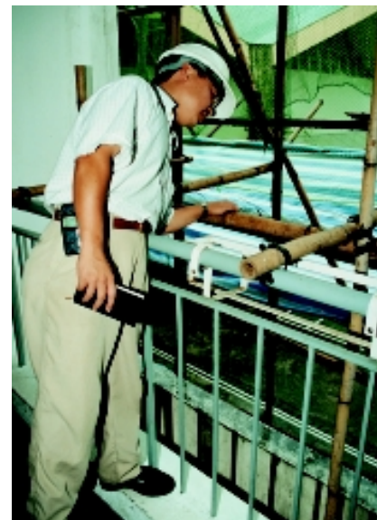
The Site Agent is conducting safety inspection
